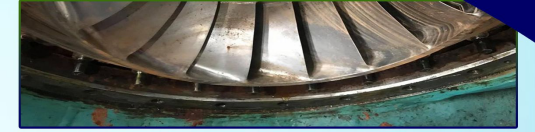
Deforme olmuş çark / Deformed Wheel
